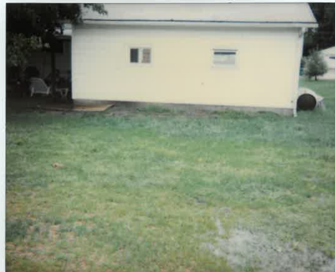
303 meekison rear yard after 2 days of morning rains @ 3" per day. 8-25-98 1 of 3
